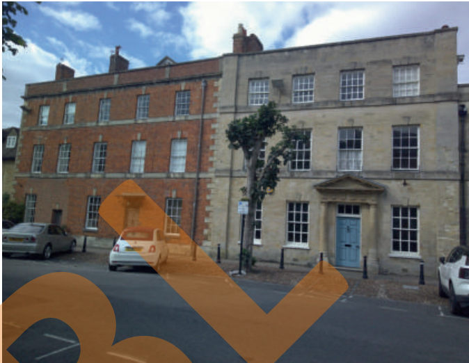
Typical Park Street sash windows
